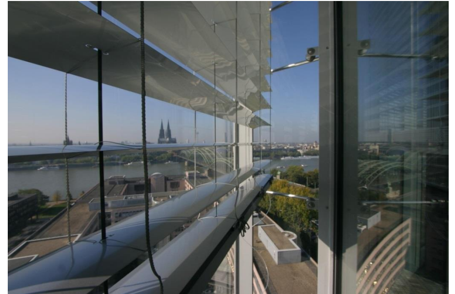
Venetian blind system mounted in the Köln Triangle building in Cologne
